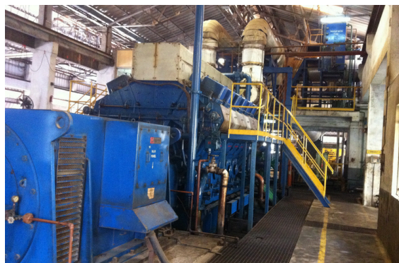
Tube Products of India, Daihatsu Generator 12DK-36
