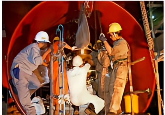
Kamome CP propeller installation
