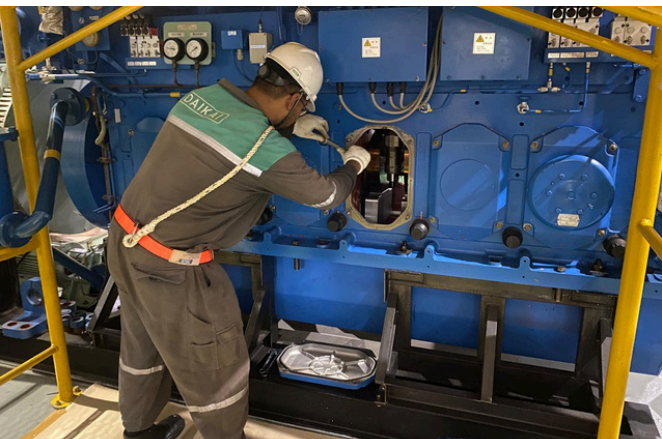
Turbo-charger overhauling
