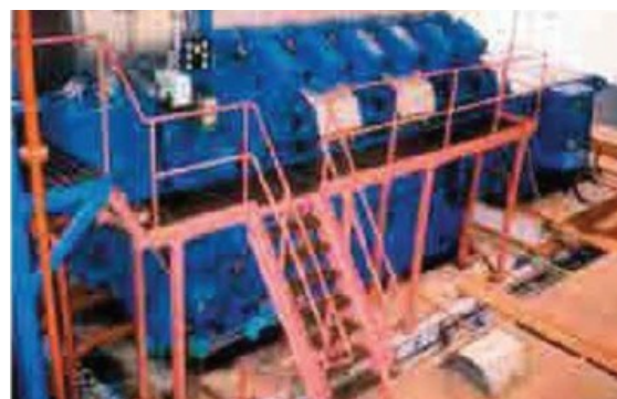
Tube Products of India, Daihatsu Generator 12DK-36
