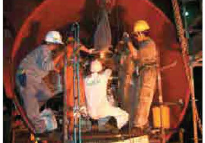
Kamome CP propeller installation
