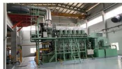
BRB Energy Limited, Bangladesh Cable Industry Daihatsu Diesel generator 8DK-36 & 12DK-36
