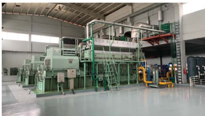
BRB Energy Limited, Bangladesh Cable Industry Daihatsu Diesel generator 8DK-36 & 12DK-36
