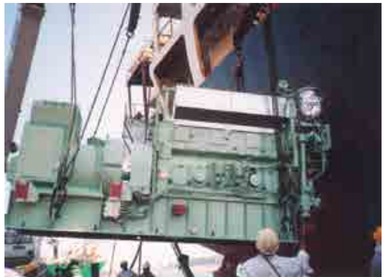
Installation of Daihatsu Engine 6DK-20 onboard the vessel Shaktidoot
