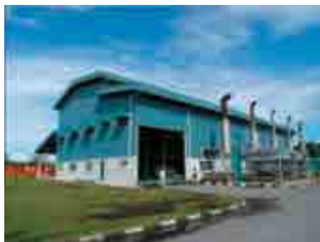
SESCO Limbang Power Station, Malaysia Daihatsu Diesel generator 12DK-32B
