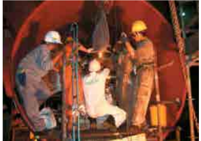
Kamome CP propeller installation
